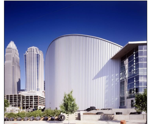
ImaginOn 's shimmering aluminum roof dramatically enhances Charlotte's city-center skyline. The energy-efficient roofing material forms the exterior of McColl Family Theater. Photo courtesy Holzman Moss Architecture
