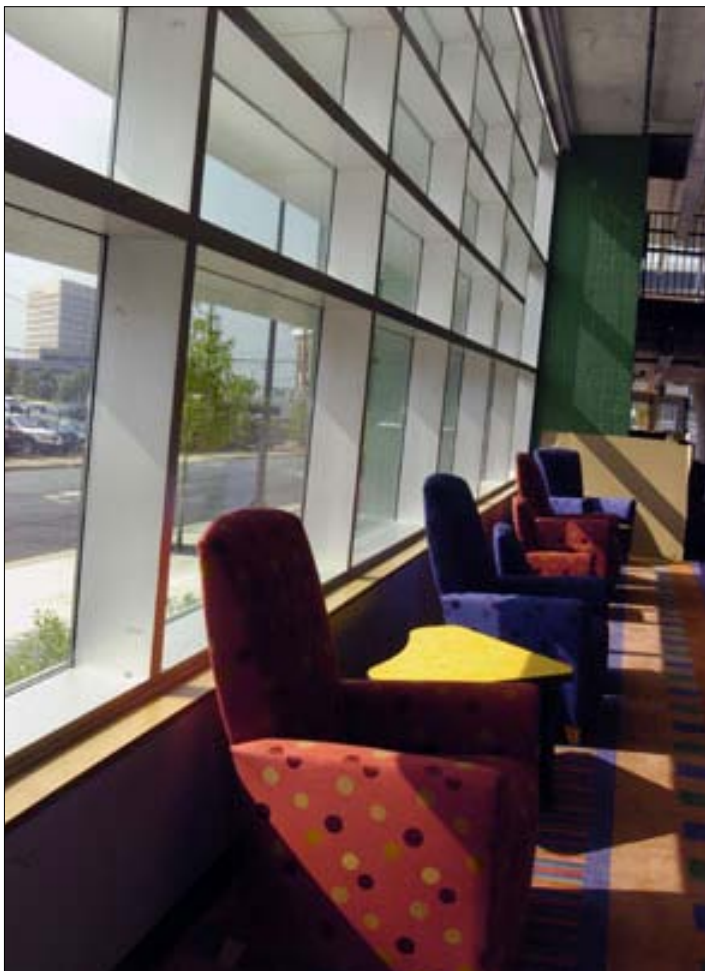
Like all the exterior walls, this one spilling natural light onto some colorful seating and carpeting is out of plumb, playfully leaning into the interior of the building.
